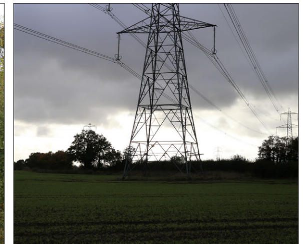
View south-west from viewpoint showing the pylons that would be removed and replaced by 400kV underground cables.
