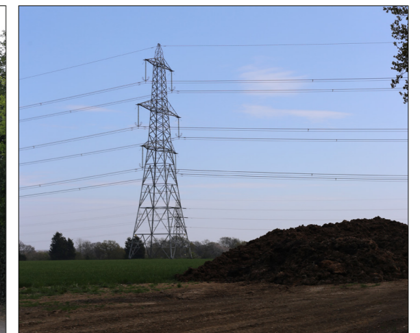
Pylon 4YL035 (photo to show full height) is in close proximity to properties in Polstead Heath and is prominent from Millwood Lane.
